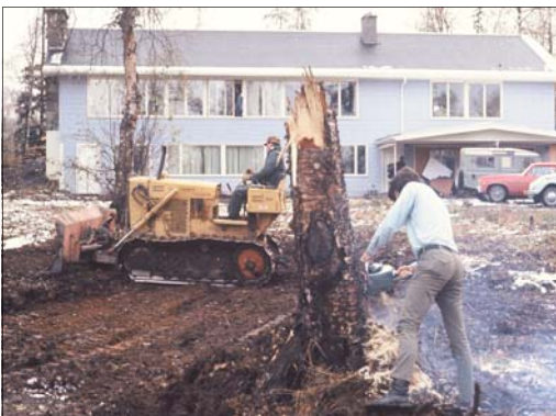
Construction in September of 1972
